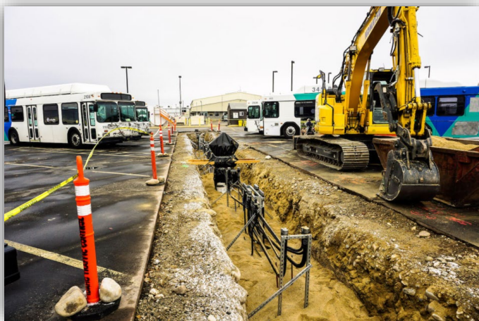
Long Runs of Trenching = Expensive
