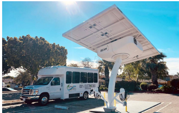
Solar Powered Charging Station
