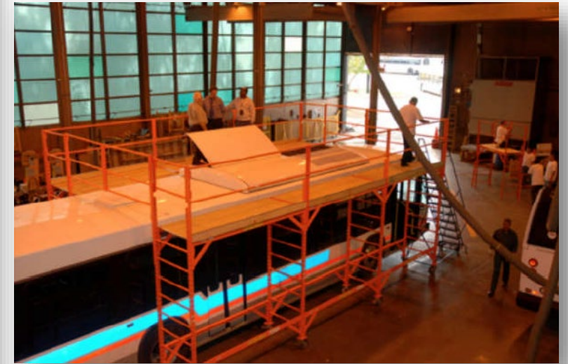
Employee Safety – Additional 10' of Clearance Between Insulated Fall Protection Work Platforms and Closest Metal Object
