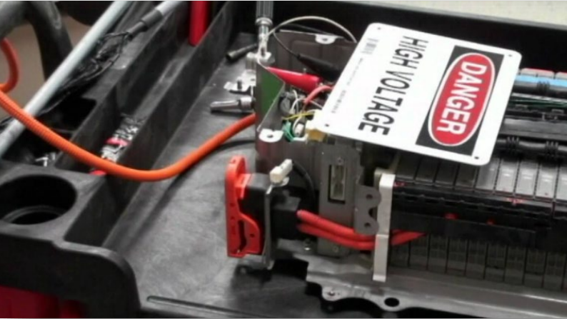
High Voltage Safety Training
